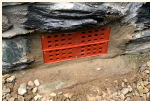
Photo: Automatically closing airbrick, Swithland
