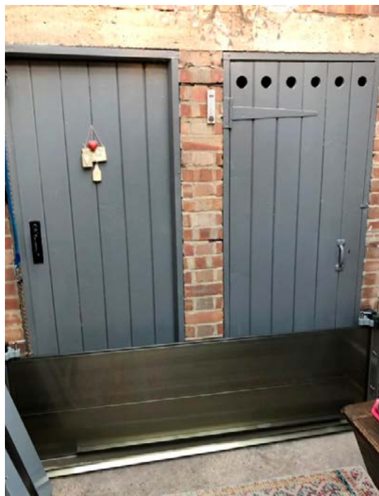
Photo: flood barrier covering two doors, Swithland
