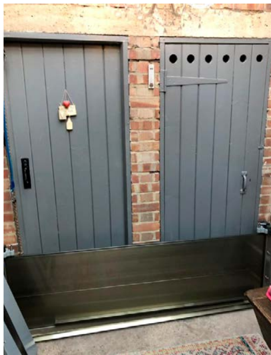
Photo: flood barrier covering two doors, Swithland
