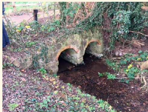
Photo: Footbridge to be removed at Breedon to increase channel capacity.
