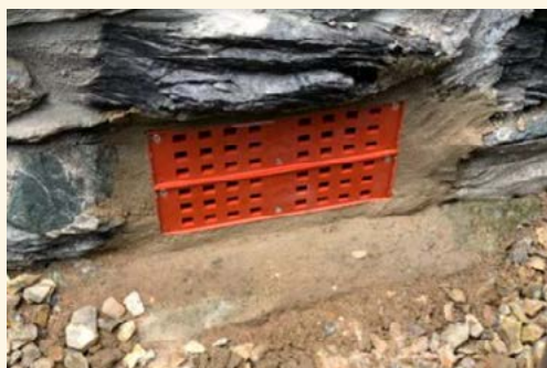
Photo: Automatically closing airbrick, Swithland
