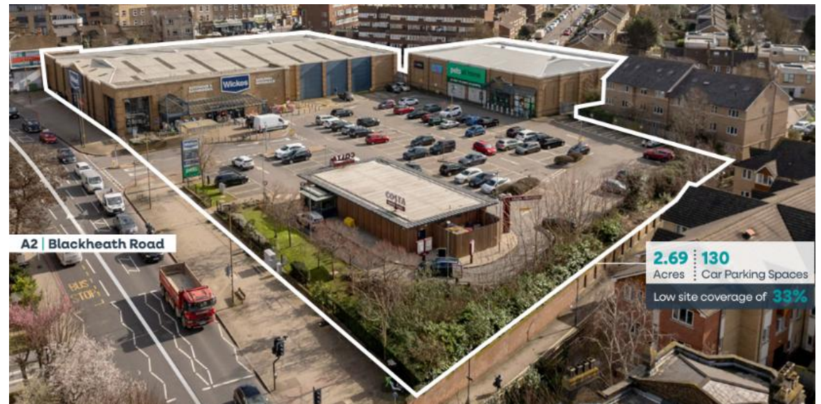
Figure: Overview of the Retail Park
