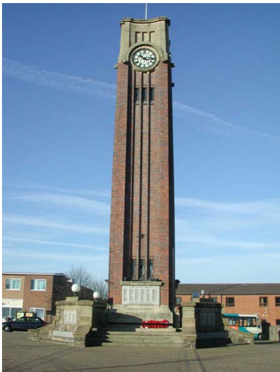
Memorial Square, Coalville, was redesigned to create public space in the town centre.
