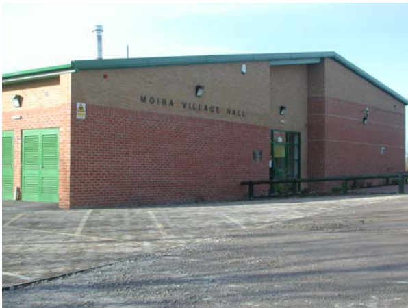
The new-look village hall in Moira
